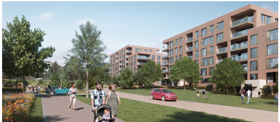
Griffith Wood, Dublin 9, achieve A2 BER rating with natural gas.
