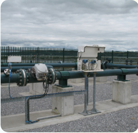
Figure 7.6: Instrumentation at an AGI
