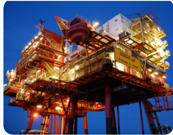
Fig 5.5: Kinsale Energy Gas Rig
