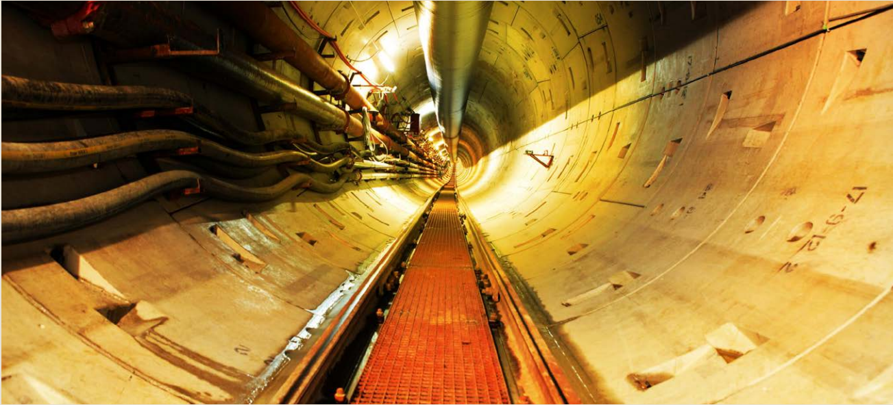
Progress on the tunnelling works at Sruwaddacon Estuary; Corrib Gas Project
