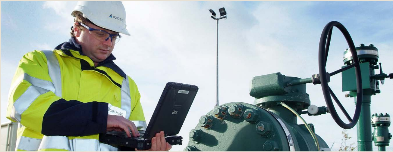
Philip Barry BGN Technician, inspecting an AGI valve
