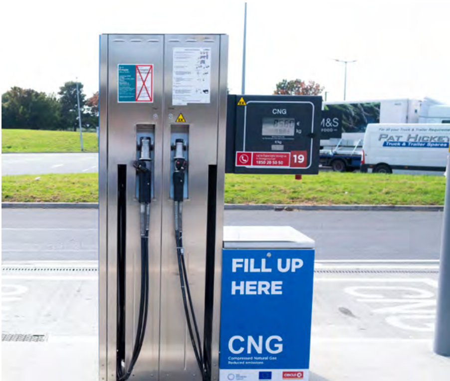
Figure 8-3: Cashel CNG station
