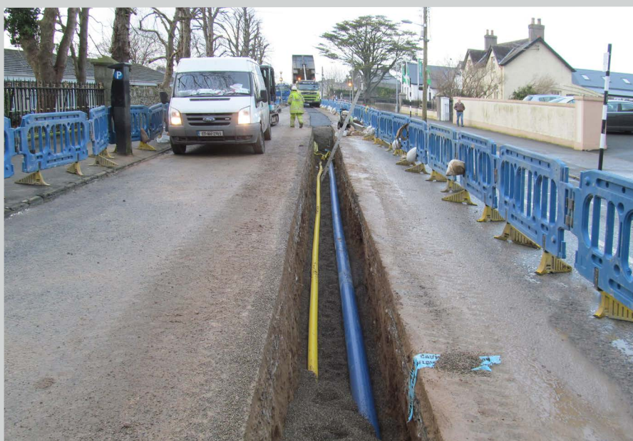
Gas and water main installation
