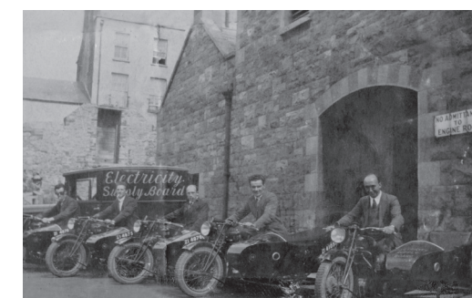
Former power generation station on Dock Road.
