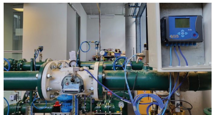
Figure 3. Volume corrector typical install
