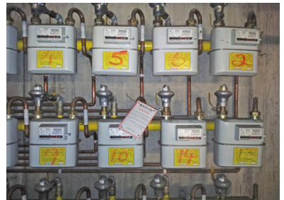
On-site meter manifold
