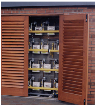
Purpose built multi-meter house (apartment complex).
