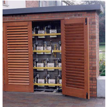
Purpose built meter manifold in purpose built meter compartment block/brick construction
