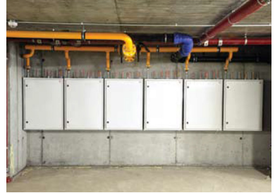
Top entry cabinet pre-fabricated off site
